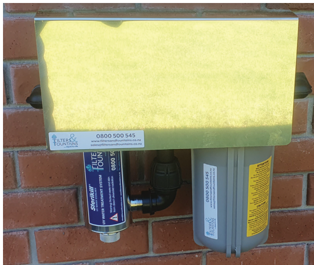
Single UV Steriliser unit - with cover (above), and (below) without cover.
